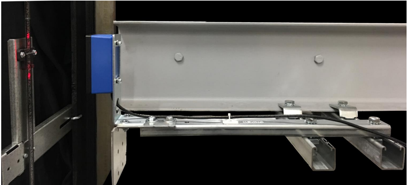
Figure E1.7: CEDES APS Camera Mounting Bracket
