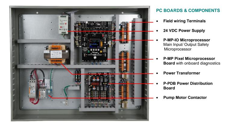
Figure 1.3.1 – Typical Pixel Hydraulic Car Controller
